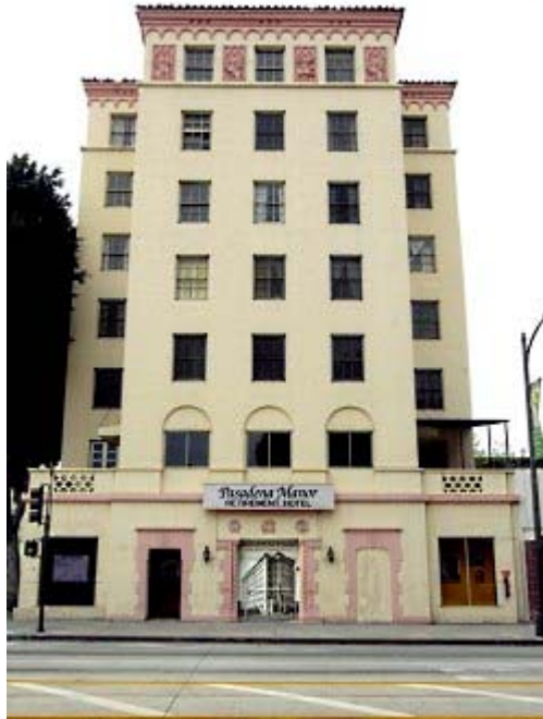
The old Pasadena Manor senior home at Colorado Boulevard and Mentor Avenue, is about to become a chic boutique hotel-back to its roots as the Hotel Constance in the 1920's. (SGVN/Staff Photo by Walt Mancini)
